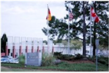
Front of Pelton & Crane
